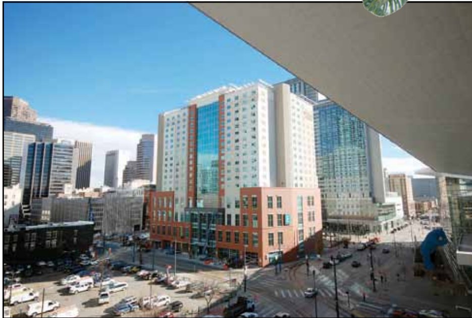
TOP: The Embassy Suites Hotel is nestled in the shadow of the Colorado Convention Center in downtown Denver. BOTTOM RIGHT: Windows had to be removed to install the 8'-0" diameter light fixtures in the lobby.
